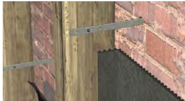
Retrofit brick ties provide a means of anchoring brick veneer to the interior stud framing during renovation. Image courtesy of Masonry Technology Incorporated.
