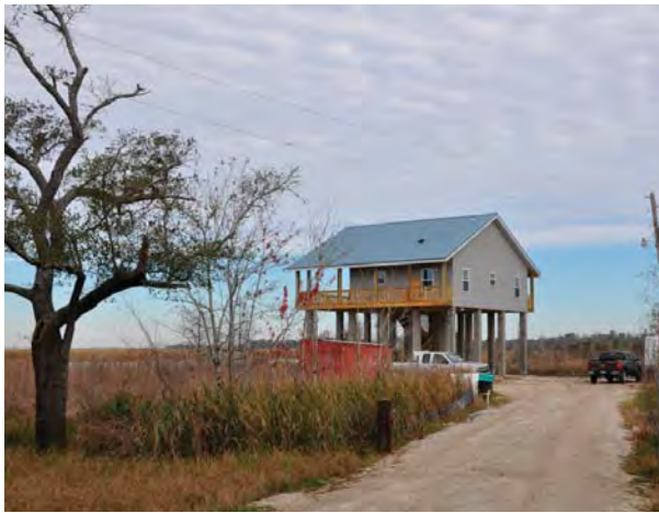
House in Pearlinton, Mississippi, that was elevated following Hurricane Katrina. Image courtesy of Gulf Coast Community Design Studio.
