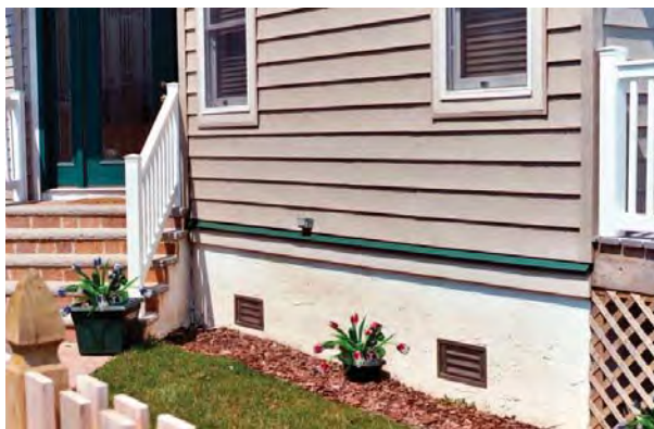
Flood openings in foundation walls are required for wet floodproofing to allow the free movement of water in and out of a structure. Image provided by FEMA.
