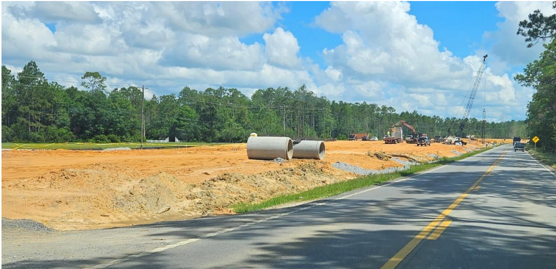
Figure 4: SR 57 Highway Construction Project
