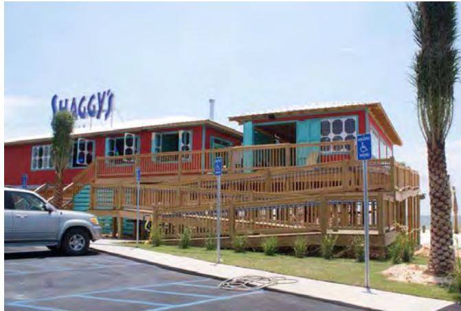
Fig. 3.2. PHOTO: Physical access problems associated with an elevated structure.
