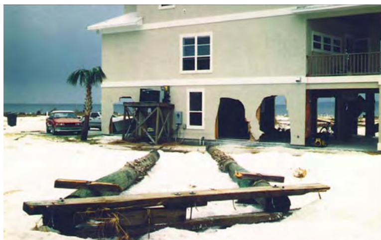
Fig. 2.12. PHOTO: Damage as a result of debris impact. ( FEMA 55 2005 )
