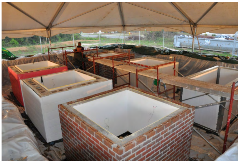
Fig. 4.3. PHOTO: Flood tank prior to flood simulation 1.
