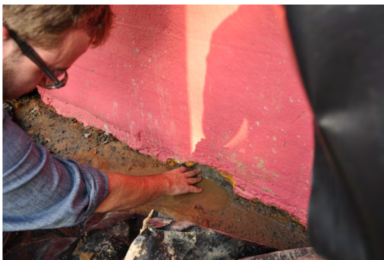
Fig. 4.19. PHOTO: Damage to test pod A: sealed block during the test fill.
