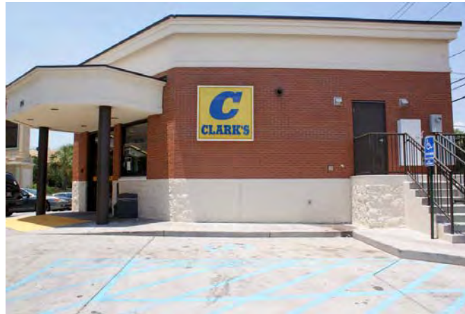
Fig. 3.5. PHOTO: Dry floodproofed structure in East Biloxi.
