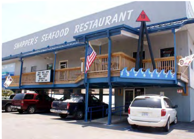
Fig. 3.3. PHOTO: Visual access problems associated with an elevated structure.
