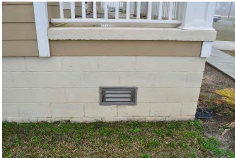
Fig. 2.2. PHOTO: Flood vent in foundation wall.
