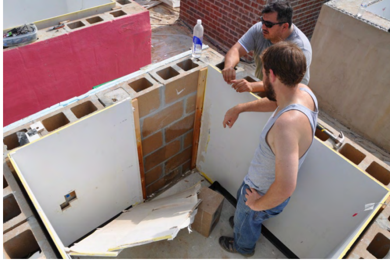
Fig. 4.5. PHOTO: Partial demolition of test pod after flood simulation.
